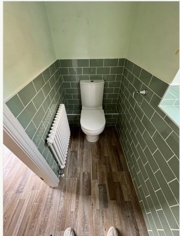
WC tiling and flooring
