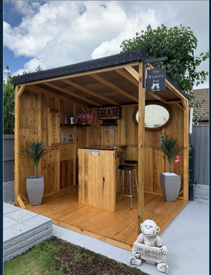
Garden structures and joinery
