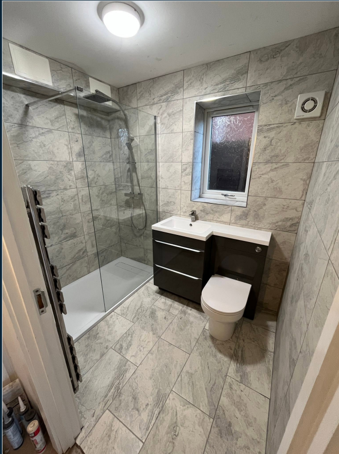
Bathroom and shower room work
